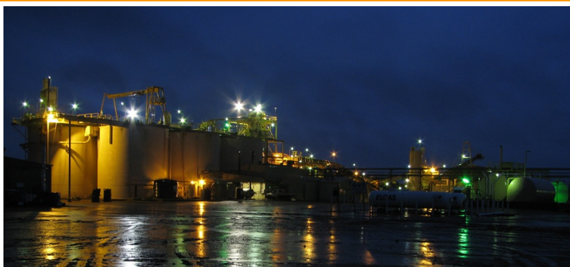
Figure 3 : 1.2Mtpa CIL Kirkalocka Gold Processing Plant
