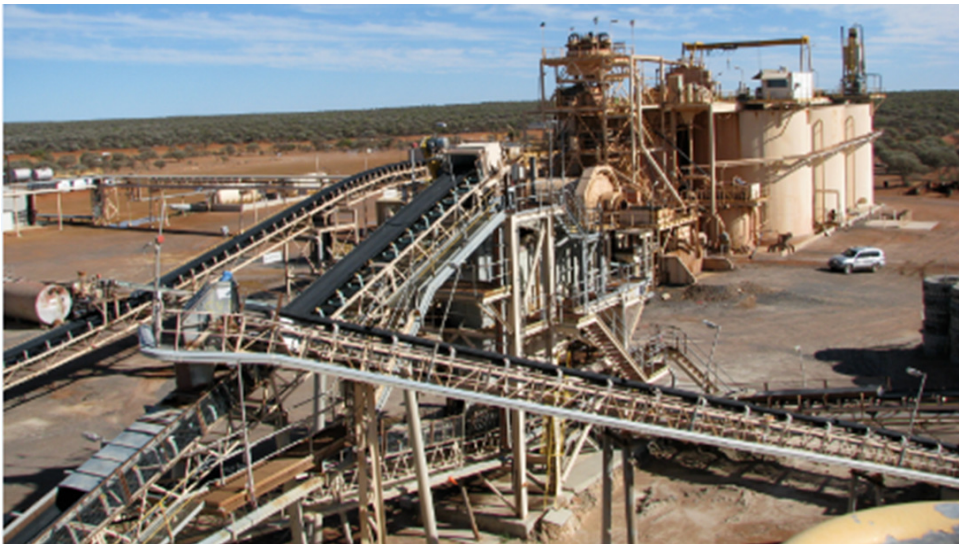
Figure 1 : 1.2Mtpa CIL Kirkalocka Gold Processing Plant
